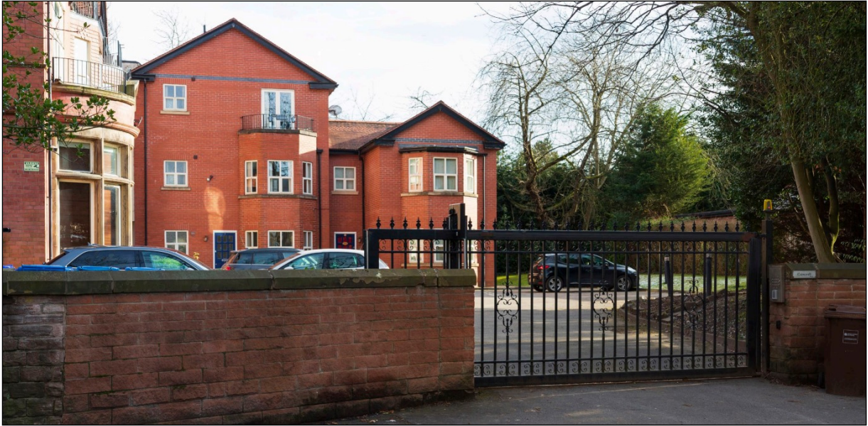
View from Holme Road of existing Cairncroft building which neighbours the site to the west
