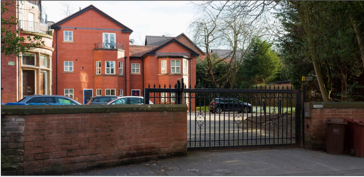
View from Holme Road of Cairncroft building with the building for the current application beyond
